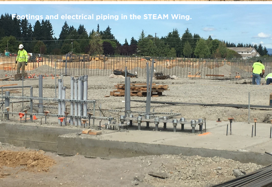
Underground work for the Main Electrical Room.
