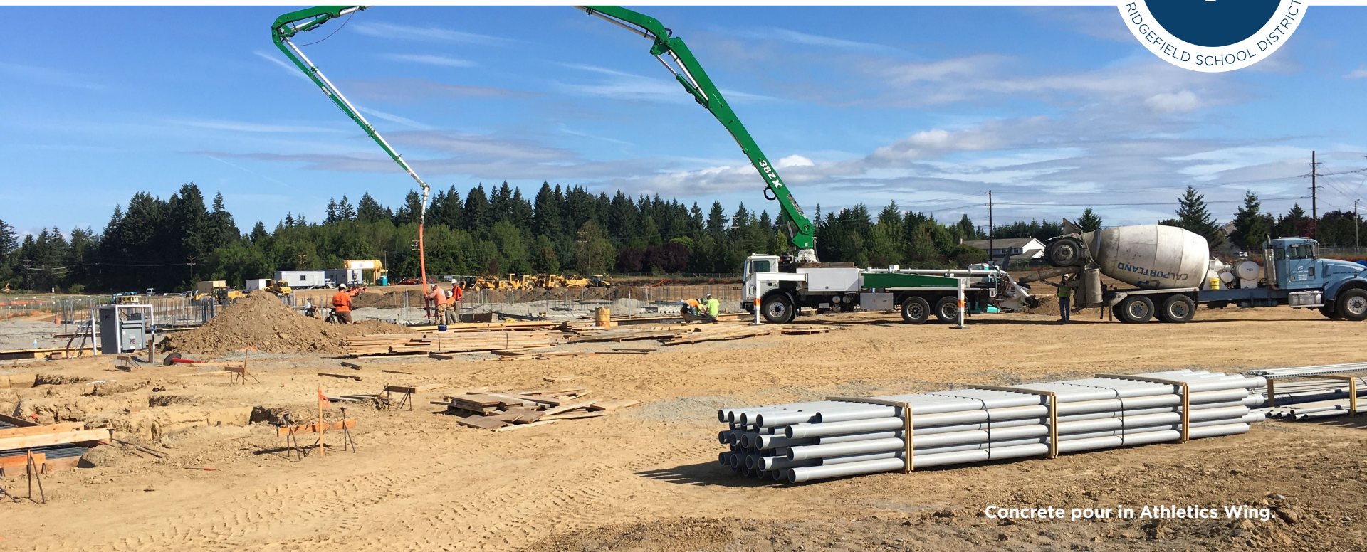
Footings and electrical piping in the STEAM Wing.
