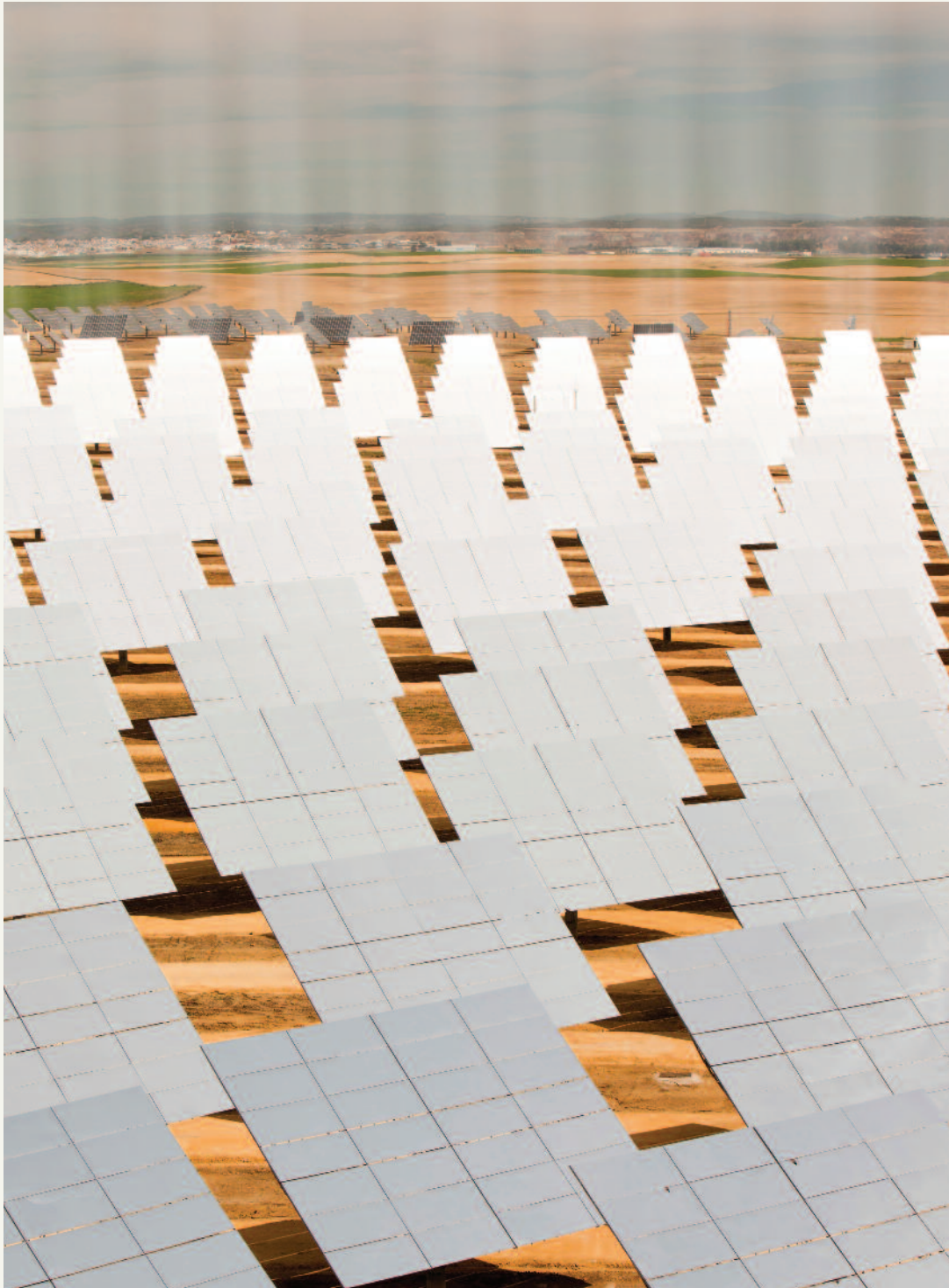
Heliostats, large reflective mirrors directing sunlight to the PS20 solar thermal tower, owned by Abengoa energy, in Sanlúcar La Mayor, Andalusia, Spain. The site generates 183 MW in total, enough to power 94,000 households and eliminating 114,000 tons of Co2 emissions annually.
