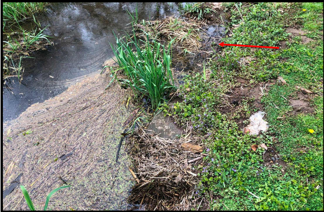
Pond inlet pipe clogged with vegetation and debris. Inlet pipe outfall into pond.
