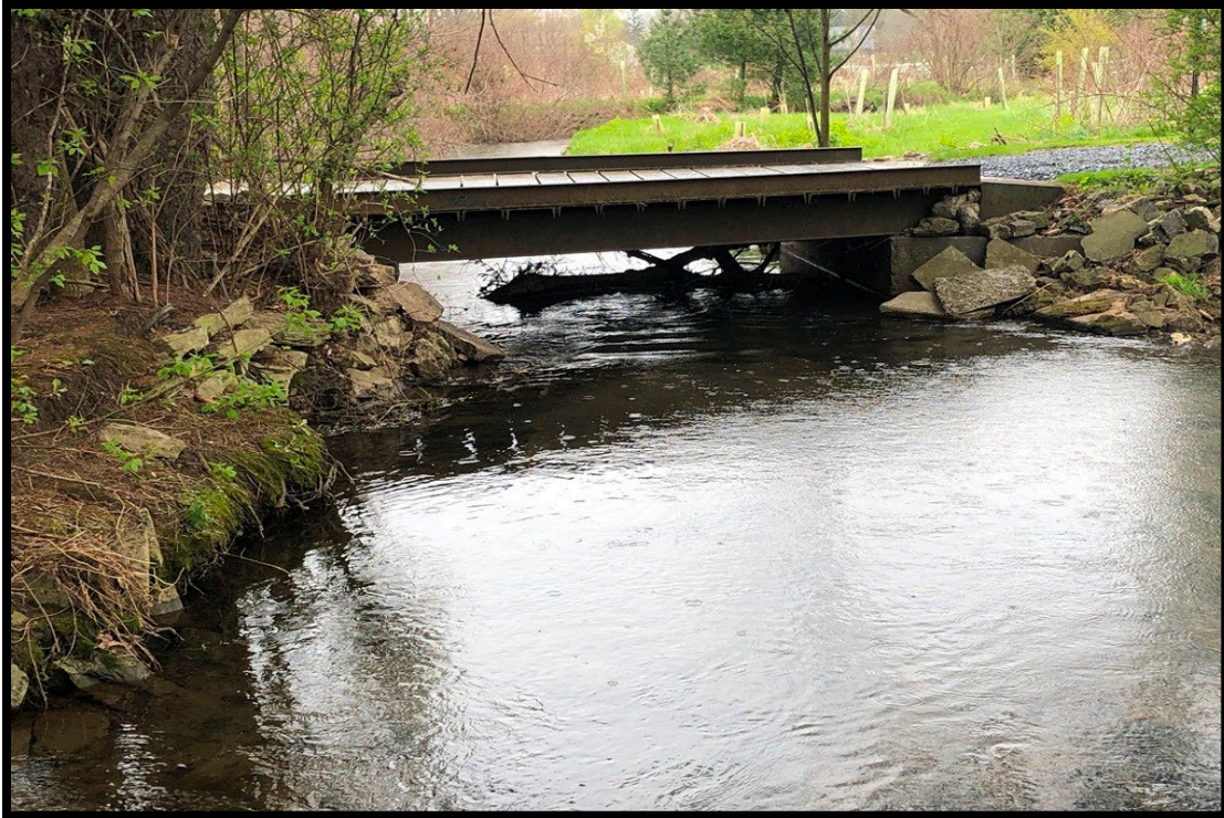
Bridge with concrete and rubble stabilizing both banks at downstream end of Reach 18
