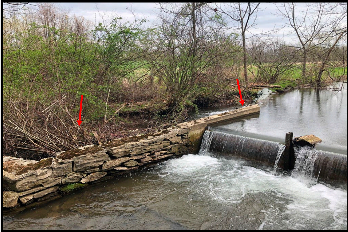
Low-head dam along middle section of Reach 18. Note eroded cutoff channel.
