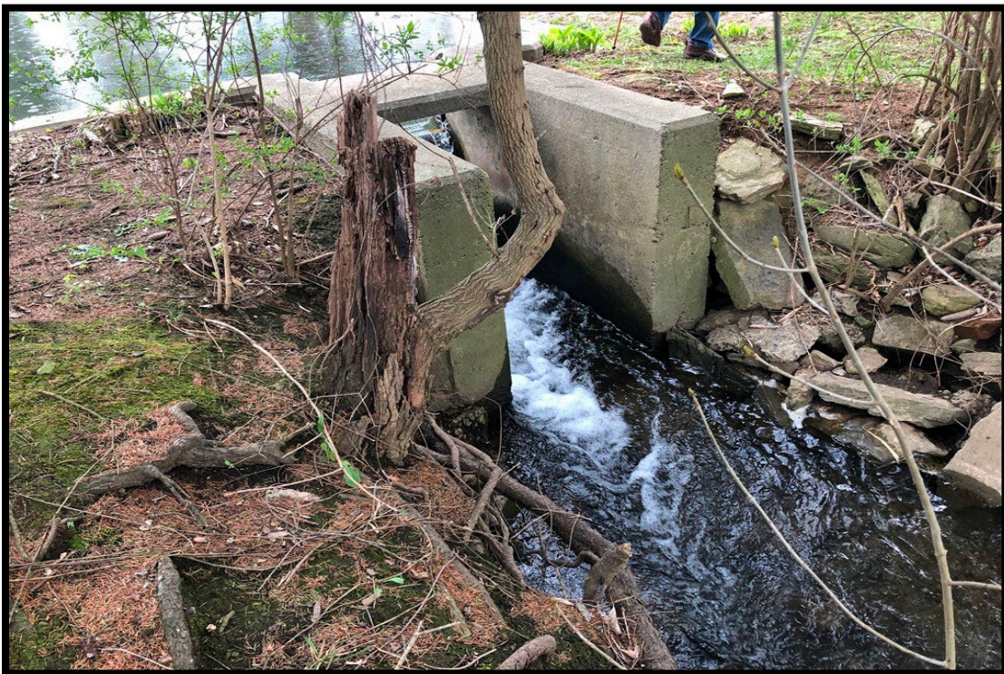
Concrete and rubble stabilizing bank eroding adjacent to pond outfall.
