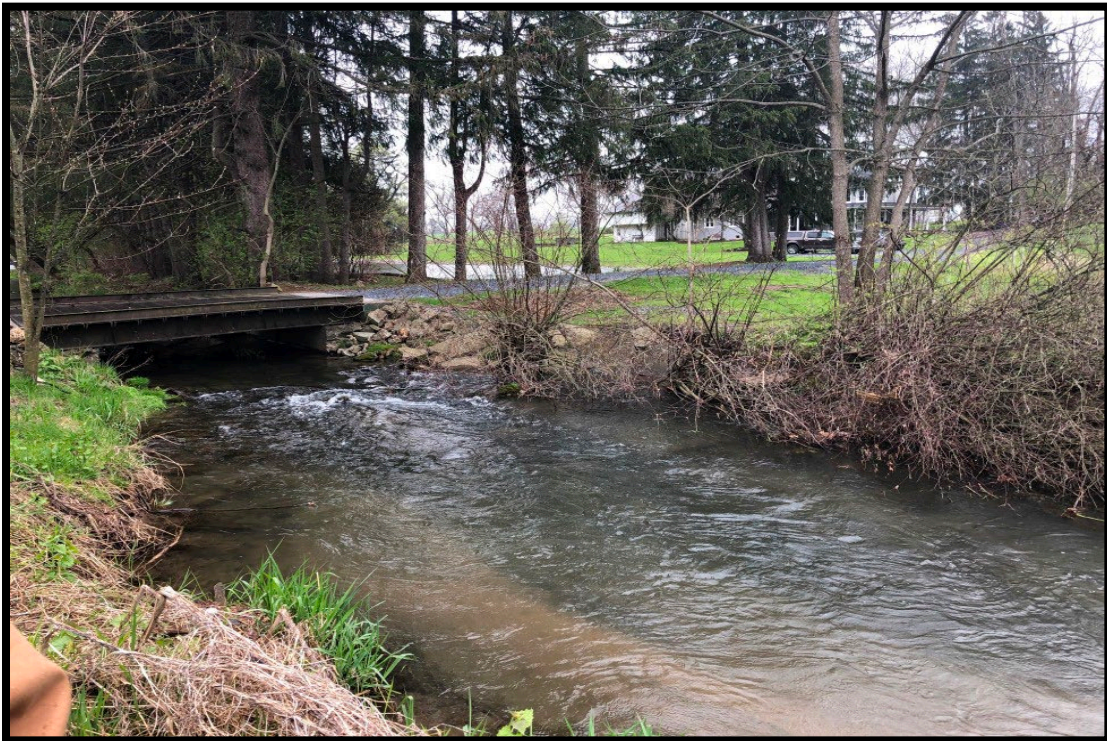
Bridge at upstream end of Reach Upper 19 with concrete and rubble stabilizing left bank.
