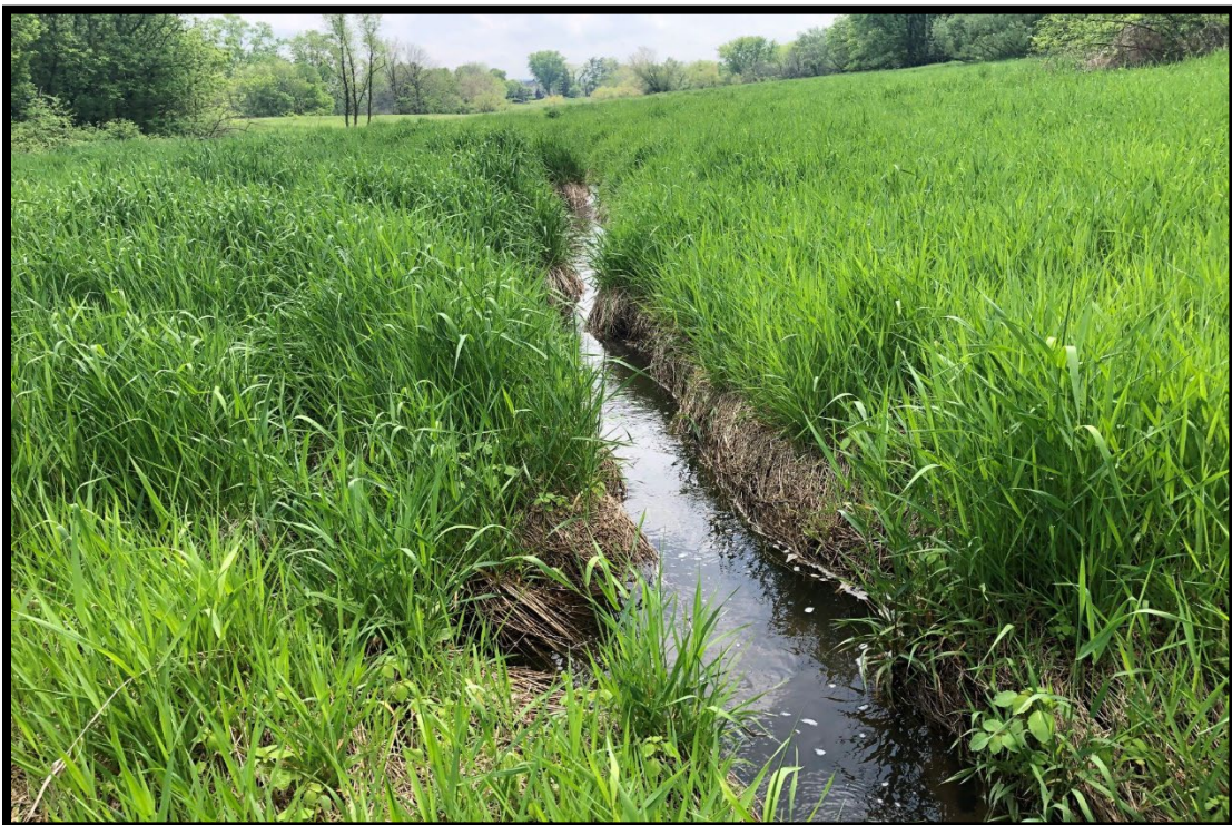
Drainage ditch evolving into eroding gully
