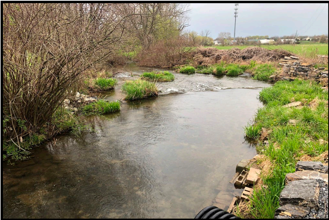
Overwide section downstream of footbridge armored with concrete, cinder blocks and rubble.
