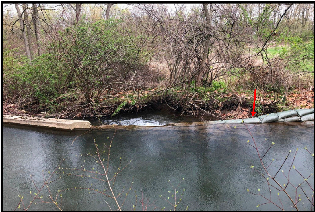
Sandbags blocking cutoff channel are temporarily maintaining the water level necessary to feed pond inlet
