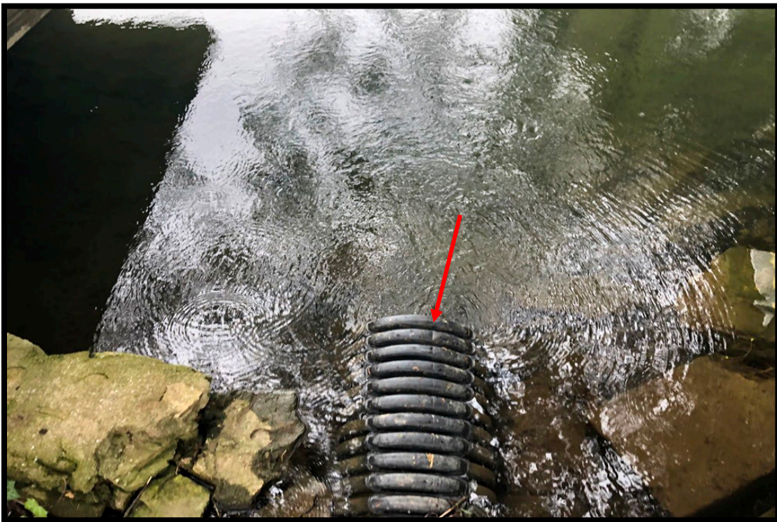
Pond inlet pipe clogged with vegetation and debris. Inlet pipe outfall into pond.
