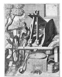
A water-powered fulling mill was later invented, with one of the earliest fulling mills in Devon established at Dunkeswell in 1238. The mechanised fulling mill brought two main innovations: first, two wooden hammers replaced human feet; and second, the hammers were raised and dropped by water power. One man was needed to keep the cloth moving properly in the fulling trough, which would have been filled with water and fuller's earth to scour the cloth and remove impurities.
