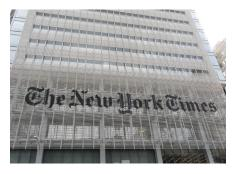
The New York Times Building in NYC (ClimAID Region 4) uses daylighting and automated shading to help improve the energy efficiency in the building. These strategies, coupled with its air distribution system, greatly reduced the energy consumption for lighting and maintaining thermal comfort. A post-occupancy report<sup>11</sup> discusses the successes of the system and some potential areas for improvement, such as individual user adjustment for controlling solar shading systems.
