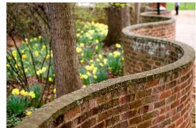
Serpentine walls at the University of Virginia approximate the shape of sine (or cosine) curves.
