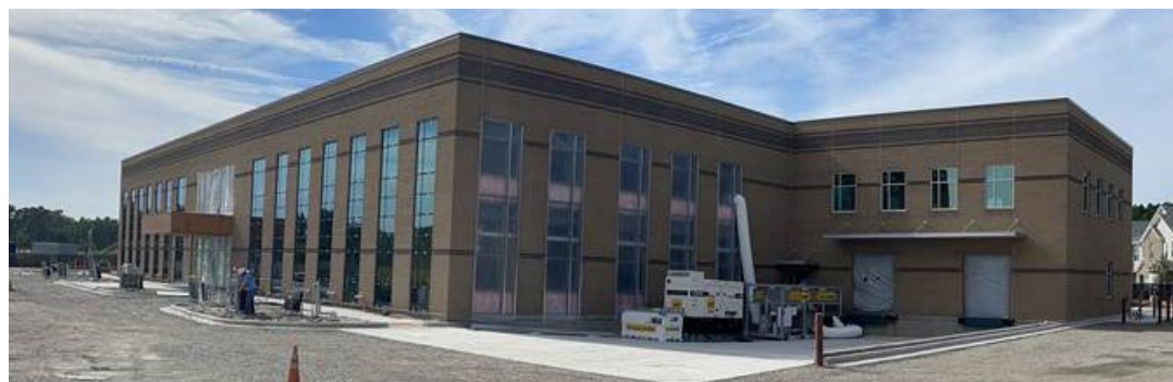
New 45,000 sq ft facility built by Environments Unlimited Inc. will support Cygnus' expansion and bring more employment opportunities to Leland, NC.
