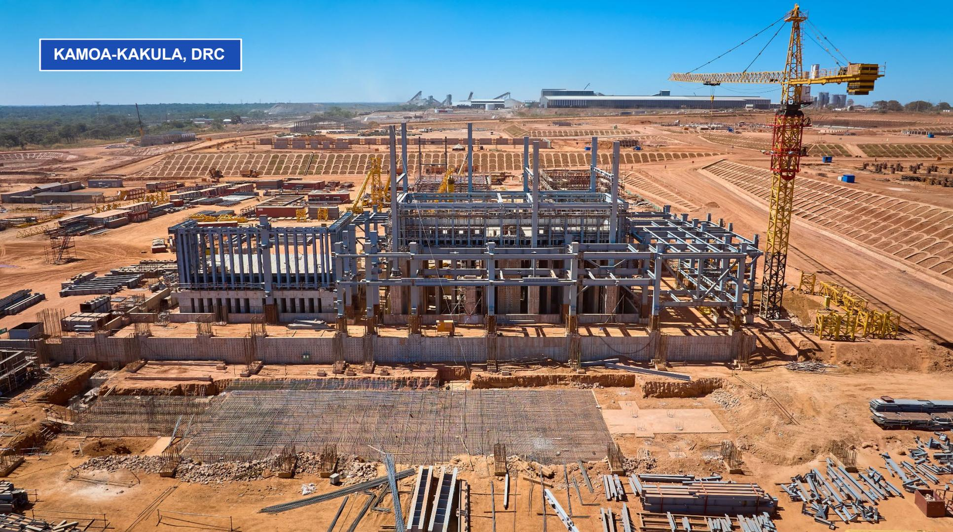
Structural steel erection is underway for the Metso Outotec direct-to-blister flash smelter furnace. The overall smelter project at Kamoa-Kakula is nearly 50% complete and is on schedule for commissioning by the end of 2024.
