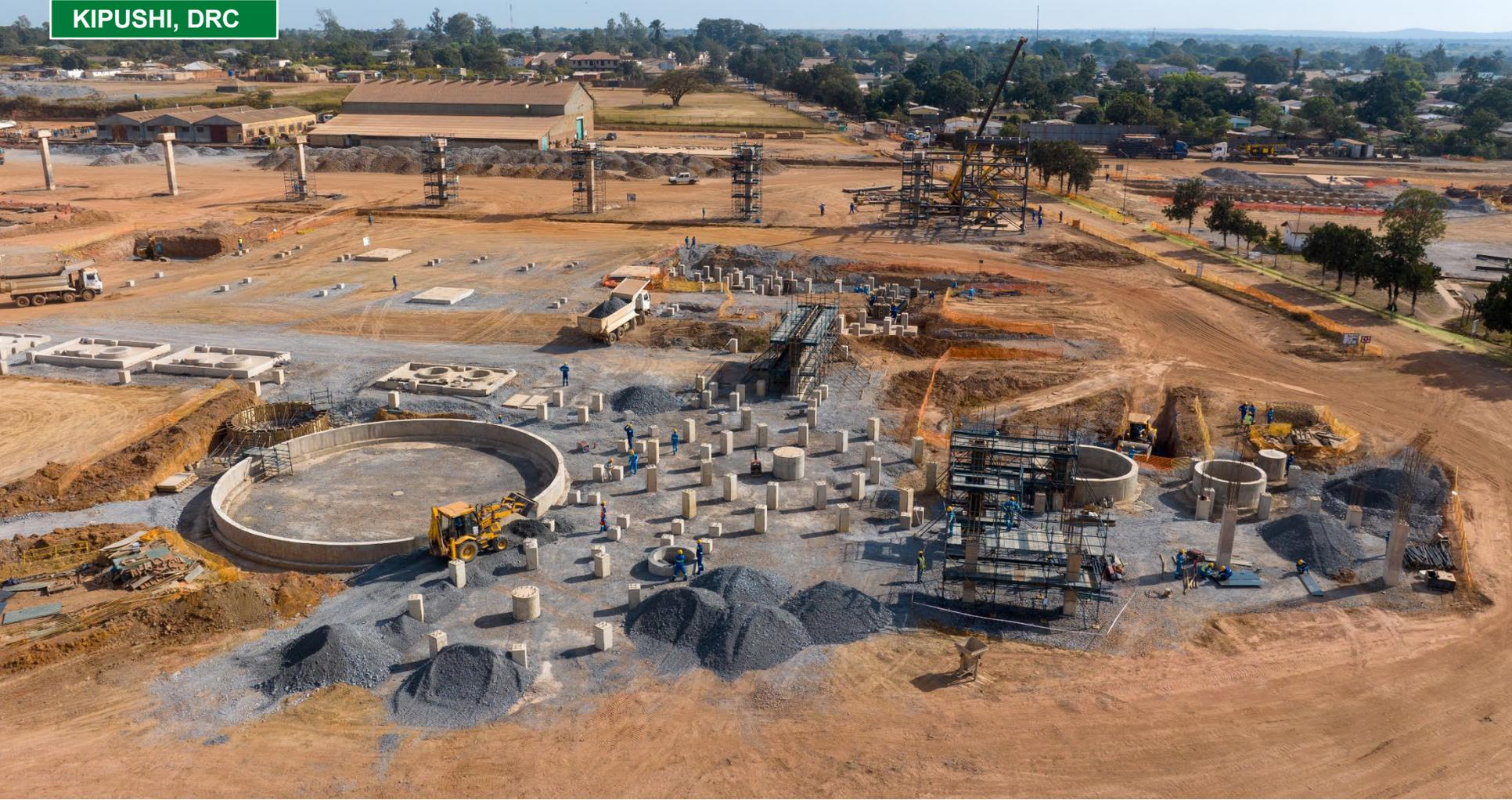
Aerial view of engineering terrace work preparation progress at the Kipushi mine. In the background are the foundations of the overland conveyor that will transfer ore from the P5 shaft to the 800,000-tonne-per-annum concentrator. Commissioning of the concentrator is expected in Q3 2024.
