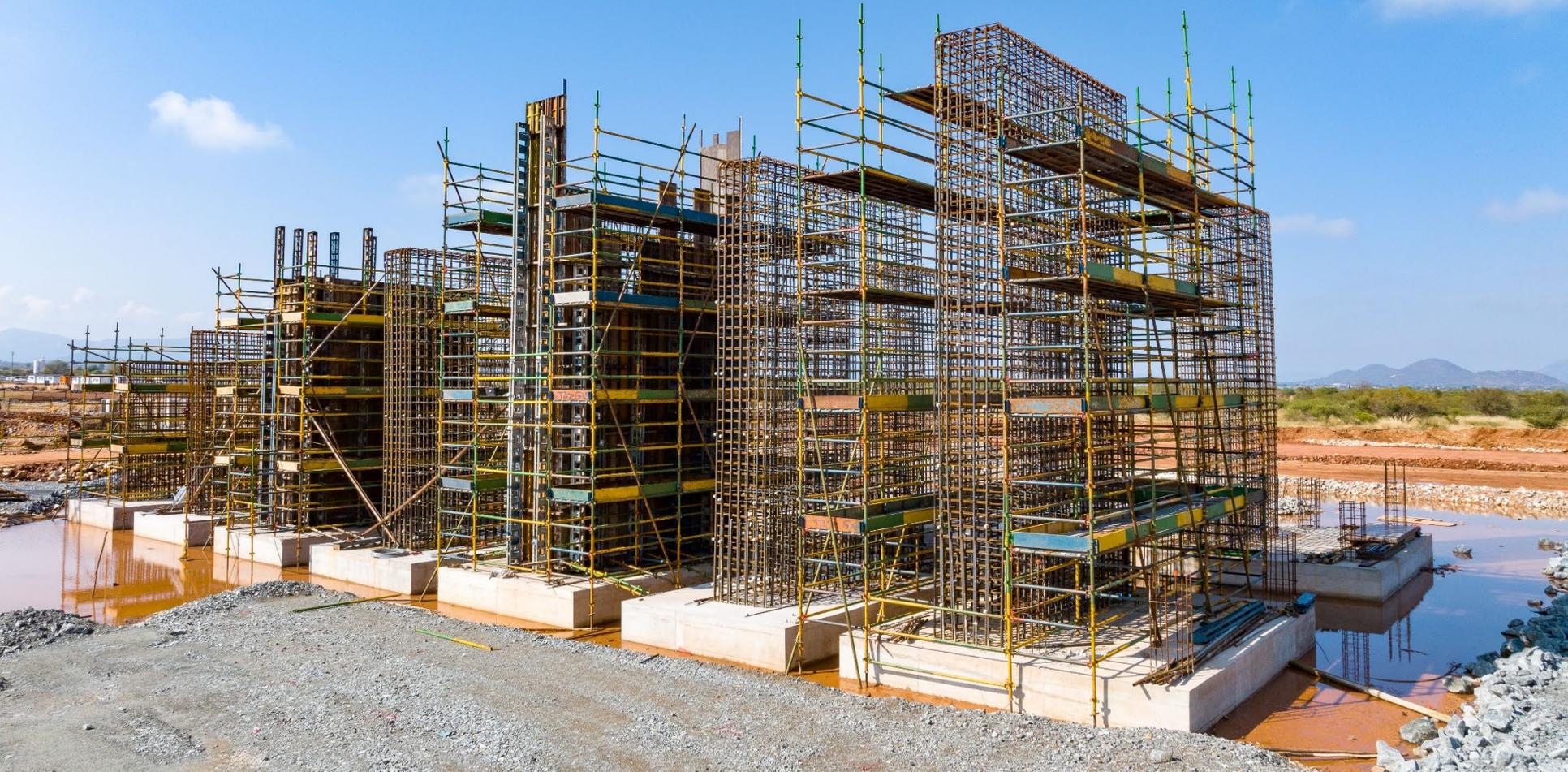
Construction of the concrete foundations for Platreef's concentrator plant flotation cells is advancing rapidly.
