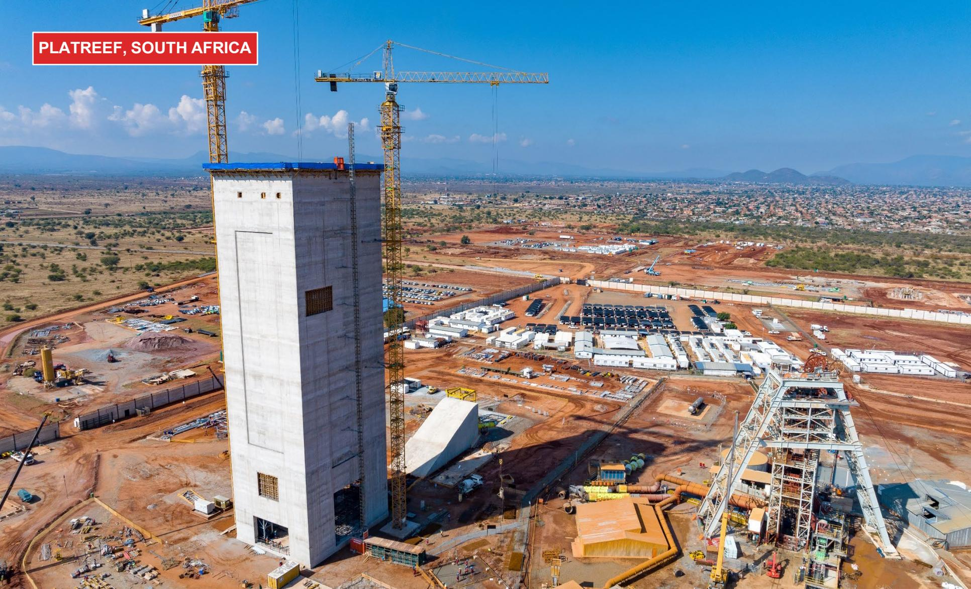
The Platreef mine site with Shaft 1 on the right and Shaft 2 on the left. The height of Shaft 2 is already 79 metres high and will reach a total height of 103 metres when complete.
