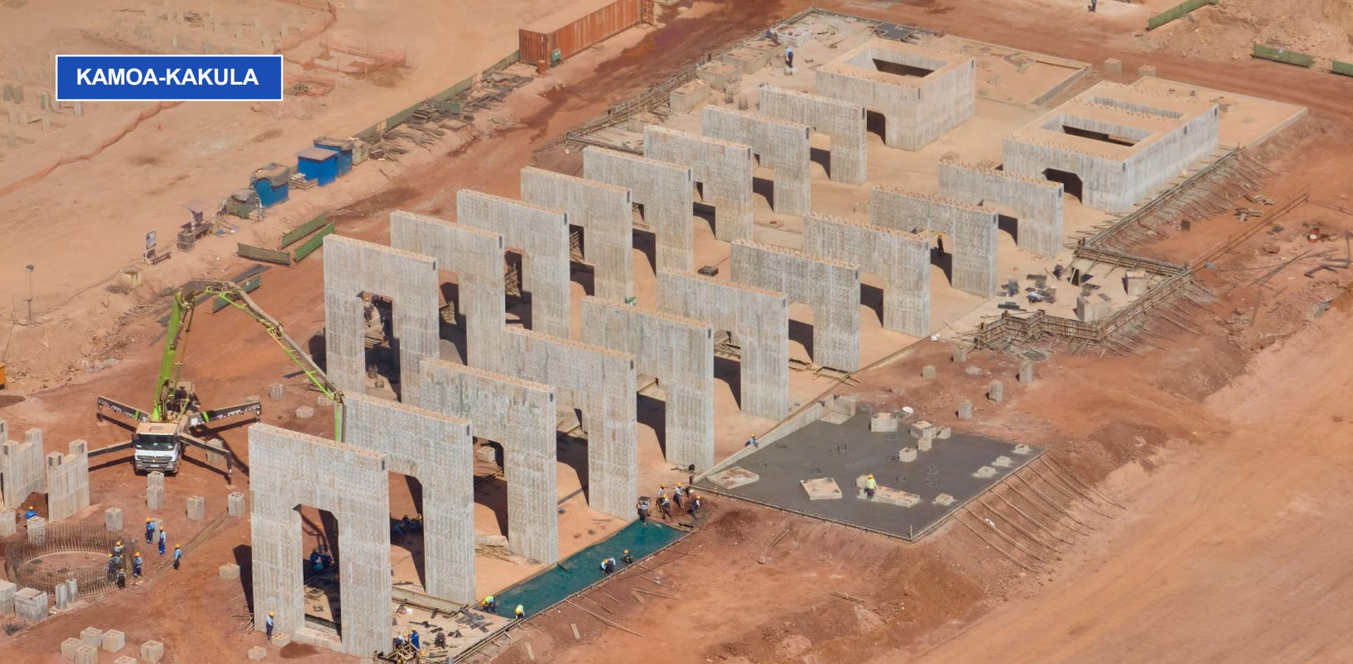
The foundations for the Phase 3 concentrator's flotation cells. Following commissioning of the Phase 3 concentrator expected in Q4 2024, Kamoakakula is projected to rank as the world's third-largest copper mining complex, with a design processing capacity of 14.2 million tonnes of ore per year and copper production of over 600,000 tonnes per year.
