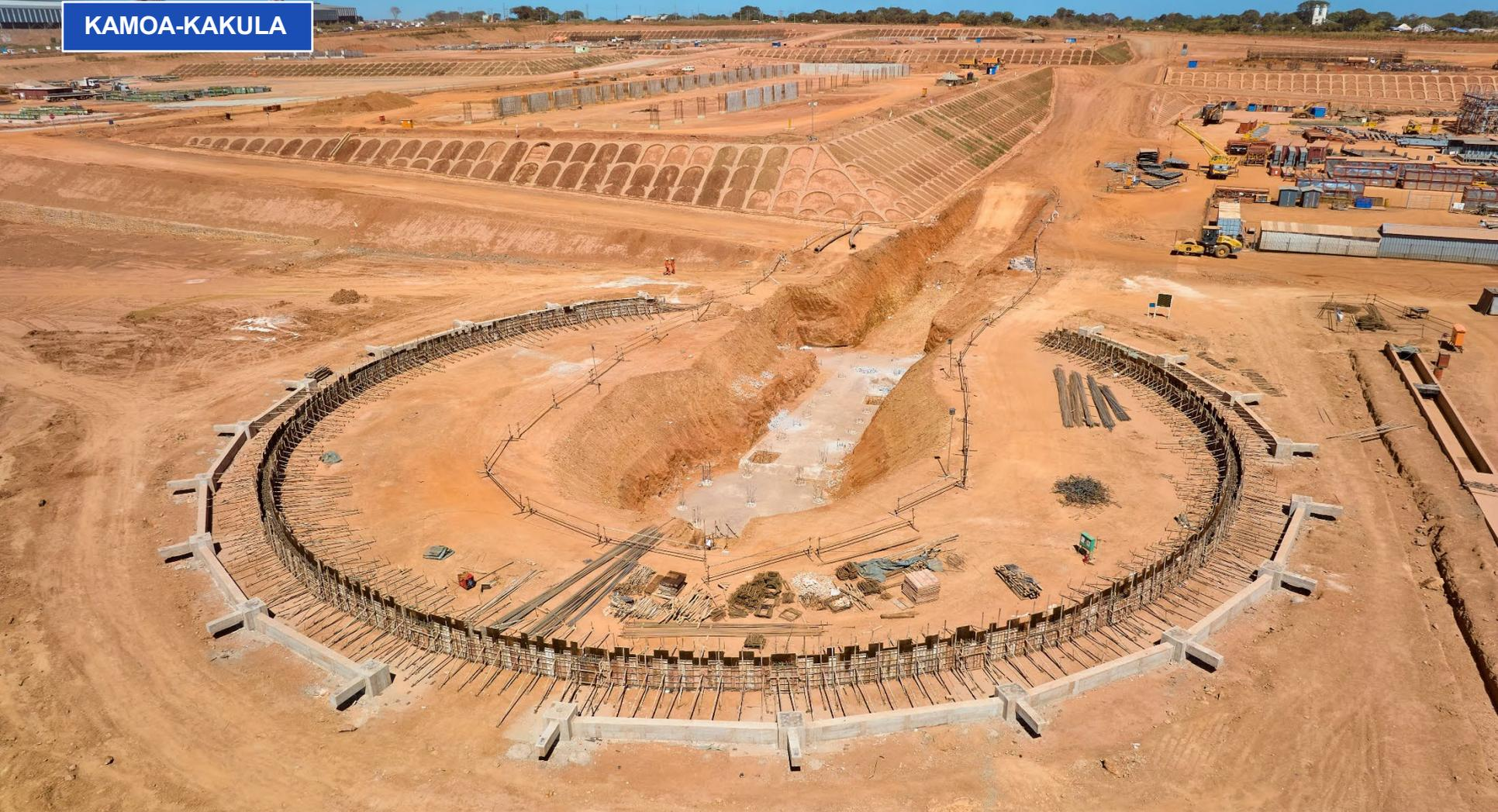
As Kamoakakula's 500,000-tonne-per-annum, direct-to-blister copper smelter complex takes shape, the concrete foundations have been cast for the concentrate-blending building (foreground).
