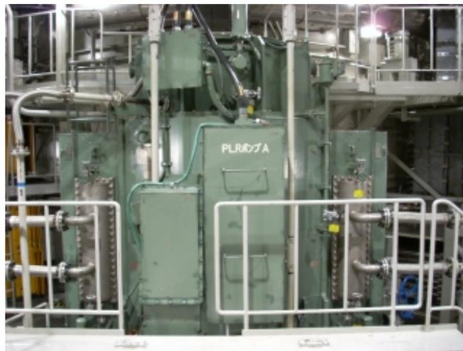
Figure 11. BWR primary coolant recirculation pump. Source: Tepco.
