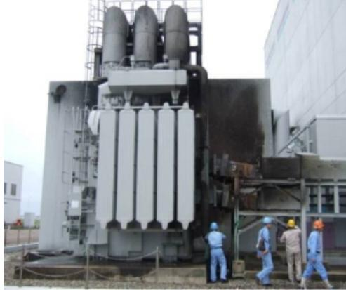
Figure 37. Transformer fire caused by 1979 earthquake. Notice the location of the transformer outside the plant enclosure and its vulnerability to water-flooding from the tsunami event.
