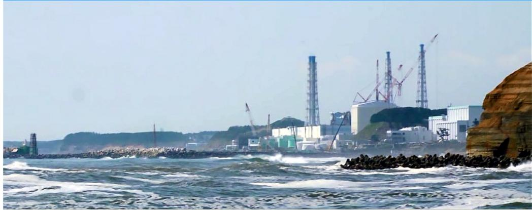
Figure 6. Siting of Fukushima plant on an artificially flattened area close to sea level. Source: Tepco.
