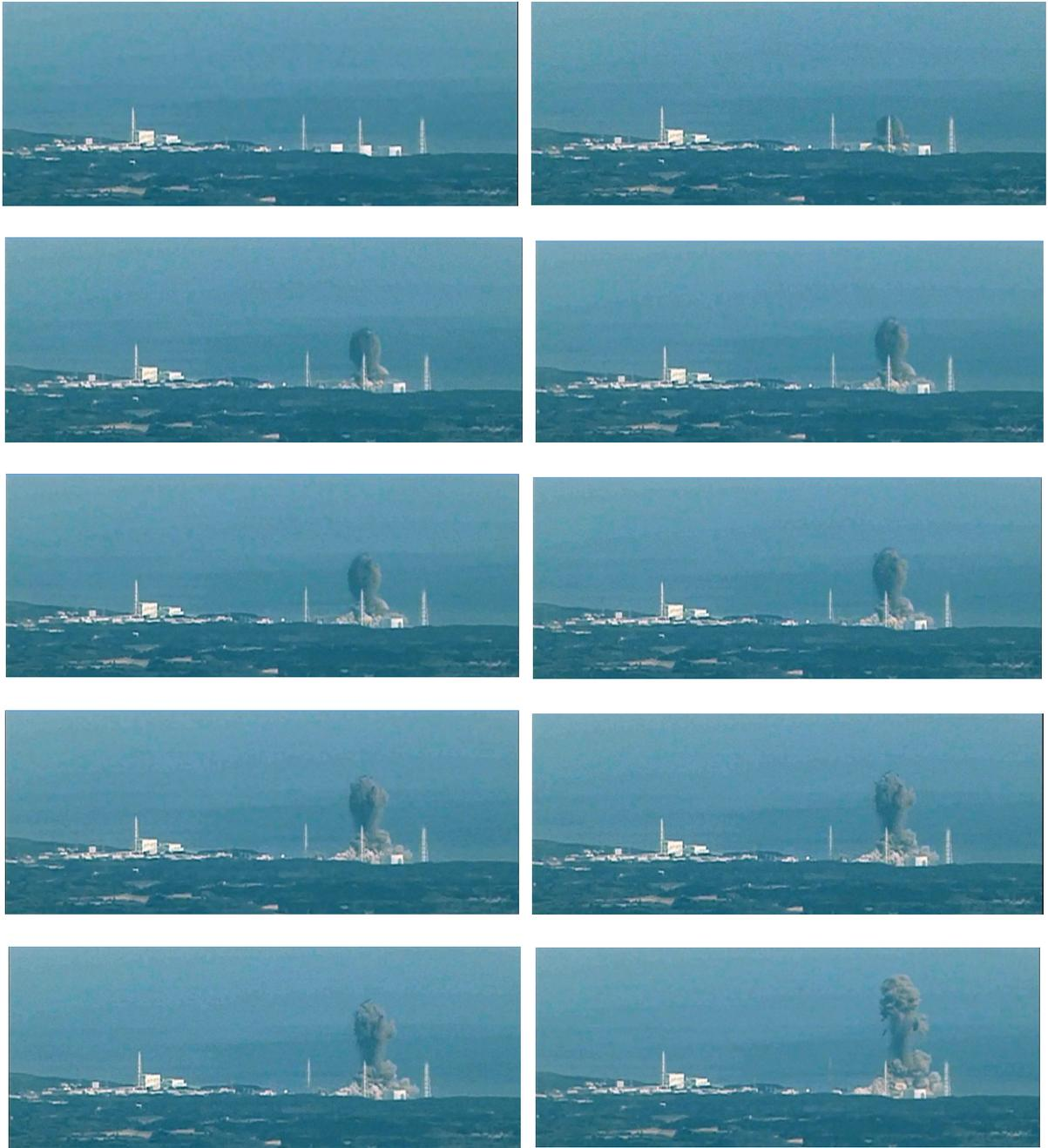
Figure 60. Sequence of vertical steam explosion following the horizontal hydrogen explosion at unit 3.
