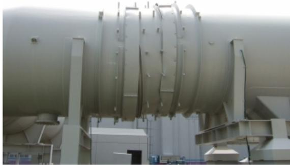
Figure 34. Earthquake-caused displacement of connecting duct to the main ventilation stack, 1979. Source: Tepco.
