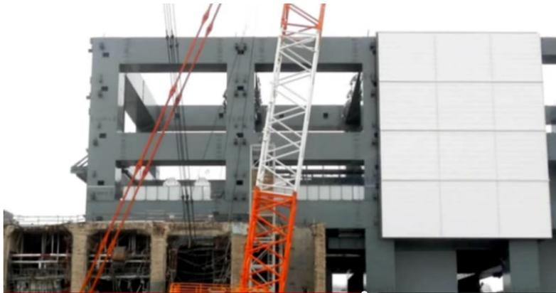
Figure 96. Adding support under unit 4 fuel pool.
