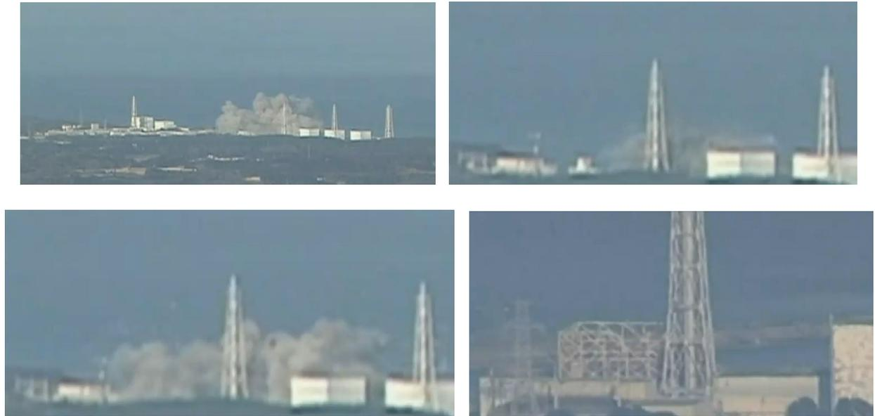
Figure 58. Fukushima Daiichi unit 1 Boiling Water Reactor, BWR nuclear power plant lateral horizontally propagating hydrogen explosion, initiated by depressurization and steam venting, sequence of events. March 12, 2011.
