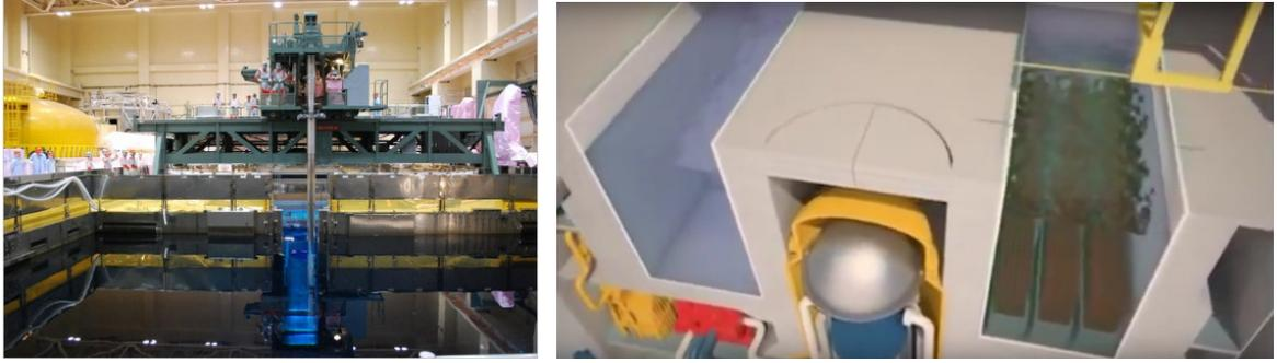
Figure 51. Refueling operation into fuel storage pool. Yellow object is the removed core dome.
