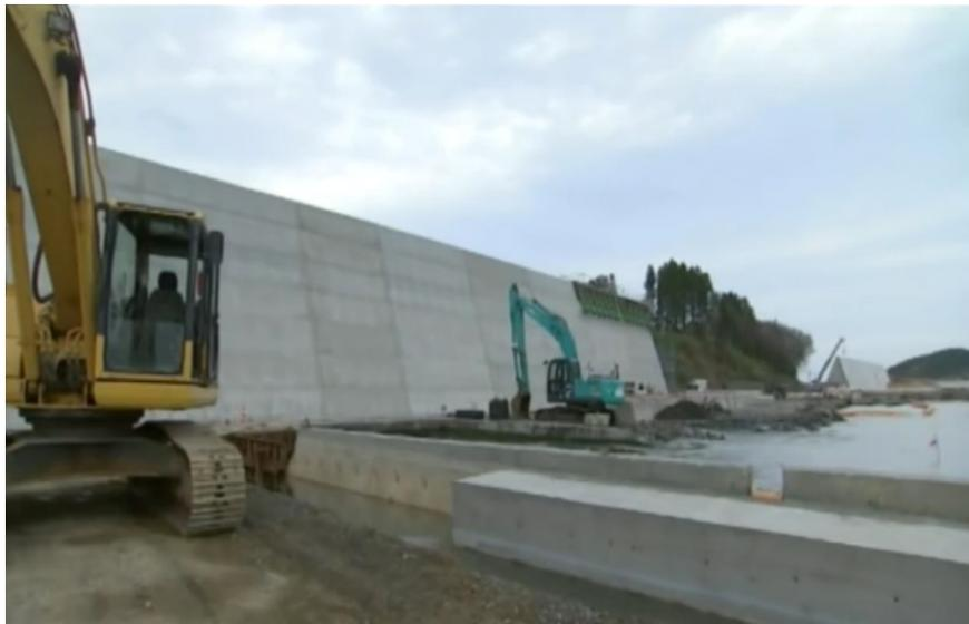
Figure 100. Concrete tsunami protection wall constructed along 400 km of the Japanese coastline.
