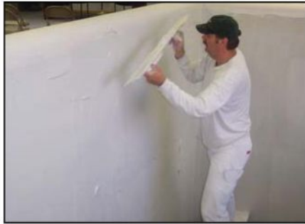
Conventional and Veneer Plaster
