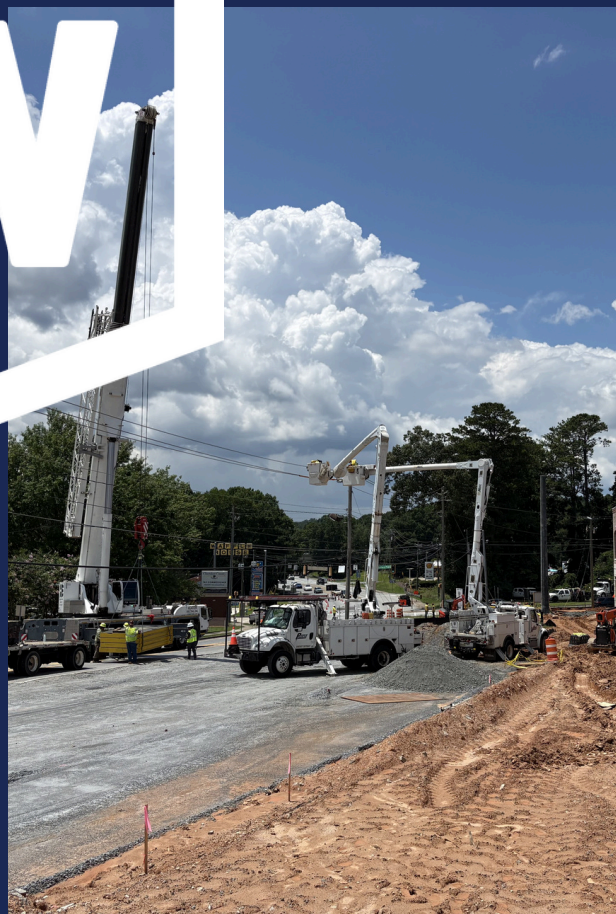
TLP - GA Power Pole Relocations
