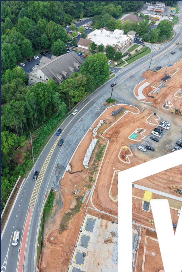
Towne Lake Pkwy Widening
